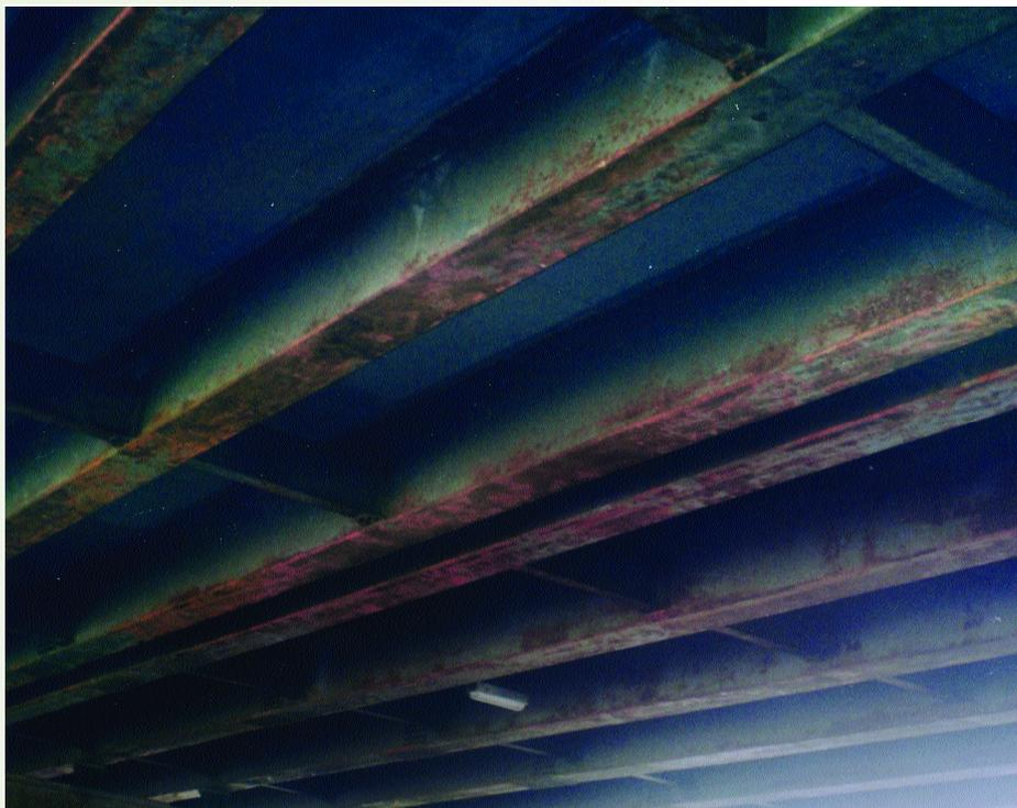
Fig. 1: Deicing salts have run down an open joint on the I-80 bridge, causing corrosion.
